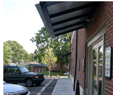
Surface parking lots should be located behind buildings or screened from street view to allow more productive uses on the street front.
