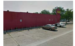
Existing: Blank walls
